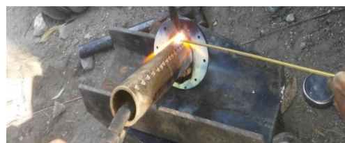
Fig. 7. Brazing of the enlarged duct with MS flange.
