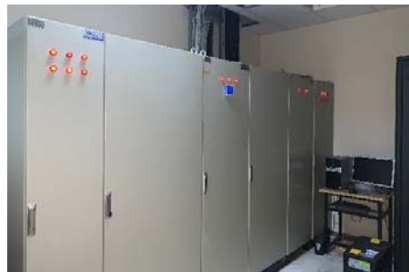
Fig. 4. Master switch cabin and cable ducts in switchgear room where fire load defined in the simulation.
