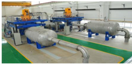
(b) Panoramic View of Pump turbine Test Bed
